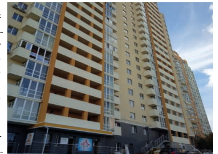
Kyiv, Novomostytskyi Housing Complex
